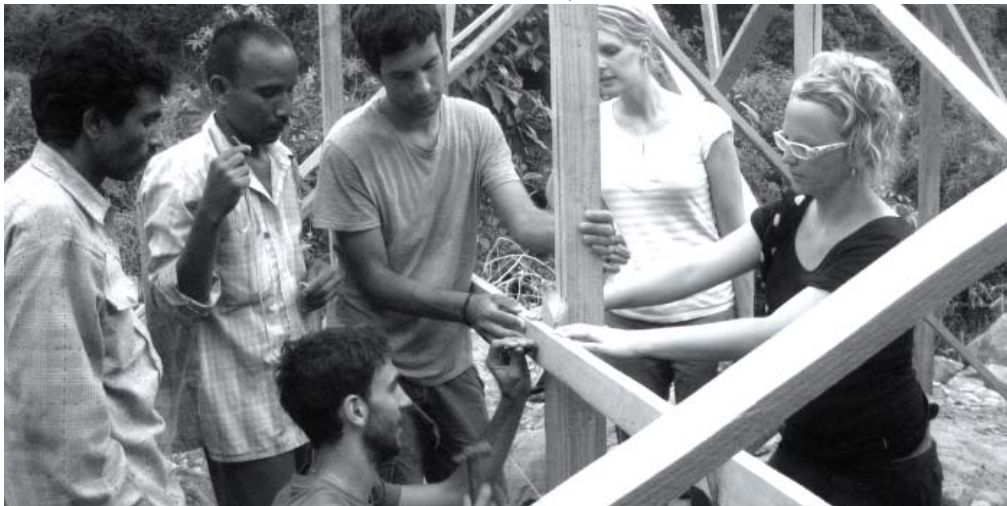
Post-seismical intermediate shelter construction in Chamoli, India
